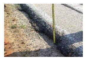
A safety edge is an inexpensive addition to a paving operation that can include a sloped drop-off which will not result in wheel catching and overcorrection errors. A 90 degree drop-off will tend to catch a tire where the safety edge slope allows the vehicle to recover to the travel way.
