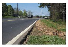
A 3 to 4-inch drop-off can easily lead to a driver "catching" a wheel off the drop-off and overcorrecting (hooking) in error resulting in crossing into head-on traffic.
