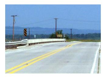
The following illustration shows a roadway with minimal shoulder approaching a narrower bridge structure with no shoulders. Object markers and guardrail were added to the approaches to call attention to the narrow structure from the road user.
