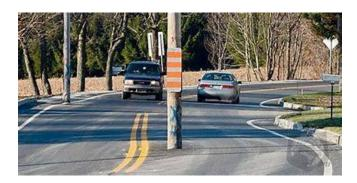
A more common occurrence is a utility pole located within the clear zone of the roadway. This often occurs due to narrow right-of-way constraints. Right-of-way can be very expensive depending on the location of the roadway and movement of certain obstruction may not be feasible.
